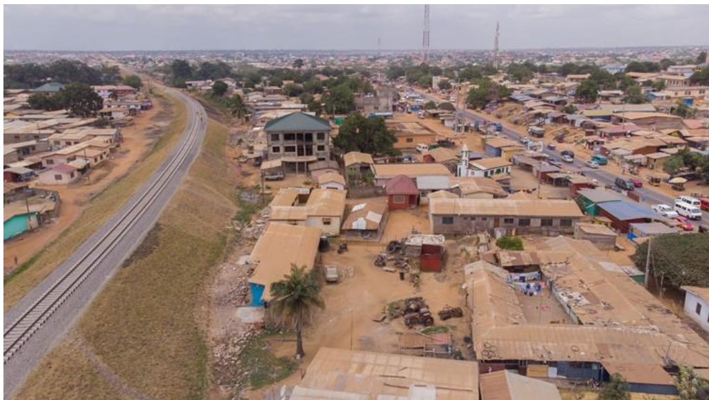
Figure 6-30 Drone capture of severance between the railway (left) and the road Specific locations for potential severance impacts are yet to be defined by INZAG.
