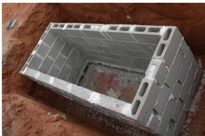
Figure 109: Individual septic tank, under construction.
