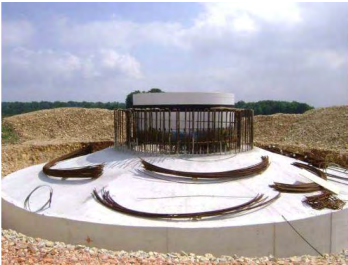
Figure 2.6 Round-Shaped Turbine Foundation
