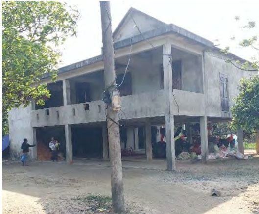
A permanent house with one-storey (stilt house)
