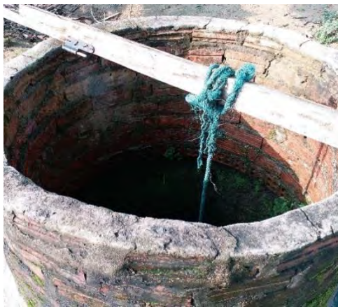
Groundwater well in Cooc village
