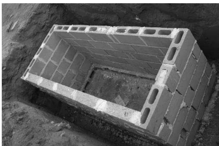
Figure 41 - Individual septic tank under construction
