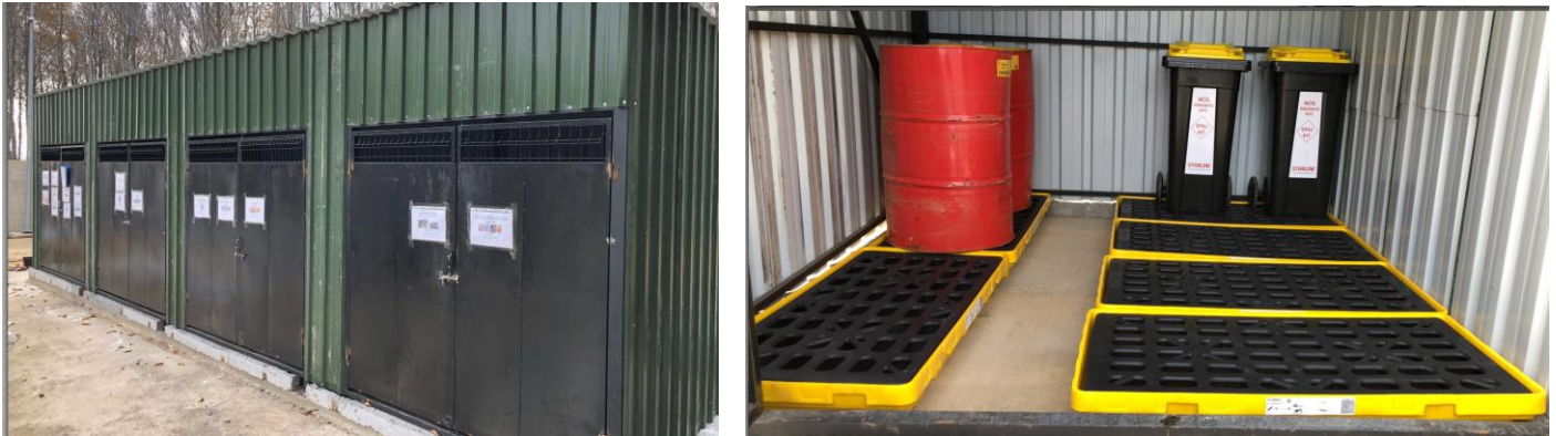
Figure 22. Waste Storage Area
