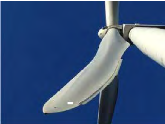
Figure 9: View of Rotor Blades
