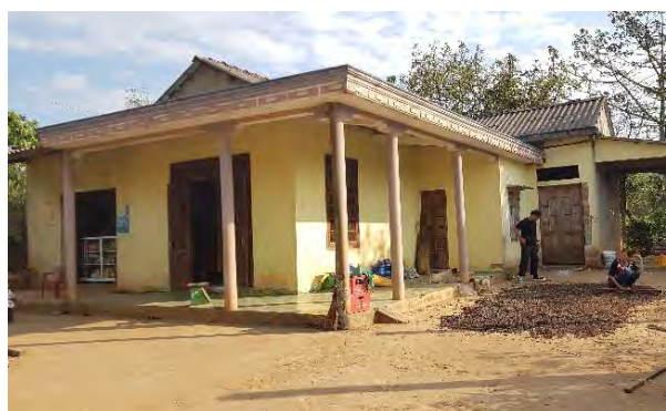
Permanent house with one storey in Cop village
