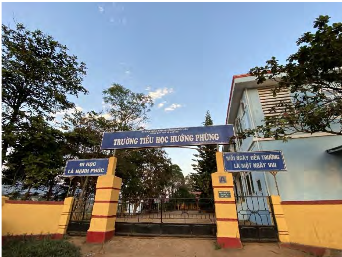
Huong Phung Primary School Located in the Commune Center
