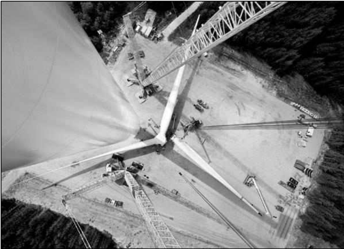
Figure I.1. Example of a Wind Turbine Platform and Installation Works
